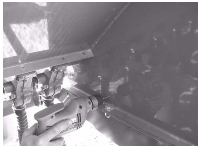
Figure 4 Drilling Pilot Hole
